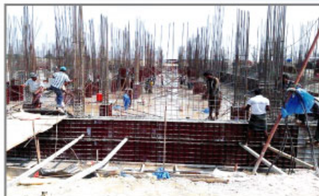
Column rebar fabrication works
