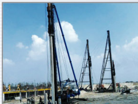
Pre-cast Pile driving works going on
