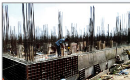
Retaining wall casting going on
