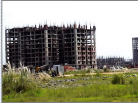
Roof casting at 9th level
