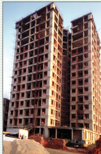
RCC framing works going on
